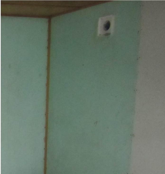
Ventilation intake plugged with a rag
